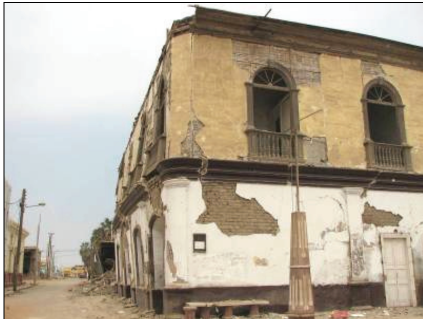
Figure 6.4 Residential building made of reinforced adobe-2
