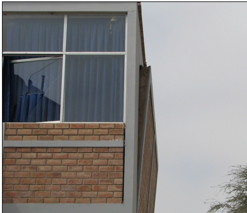
Figure 6.57 Tilted infill wall at the National University of Ica
