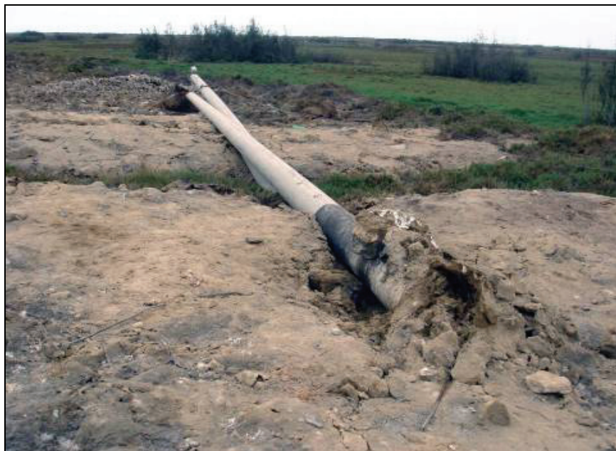
Figure 6.42 Collapse of power transmission lines
