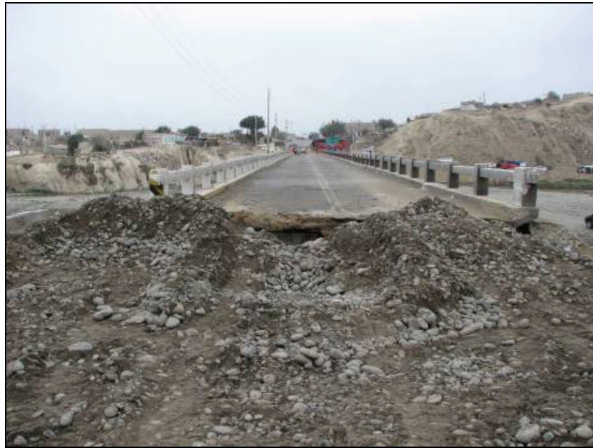
Figure 6.47 Abutment and embankment failure
