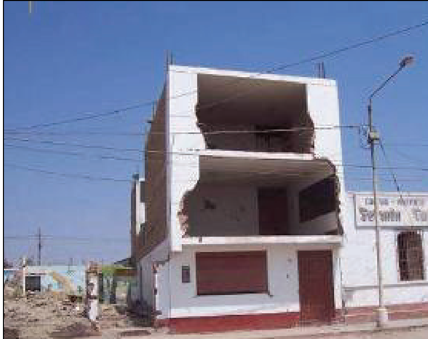
Figure 6.56 Falling of infill walls of housing unit in Pisco.
