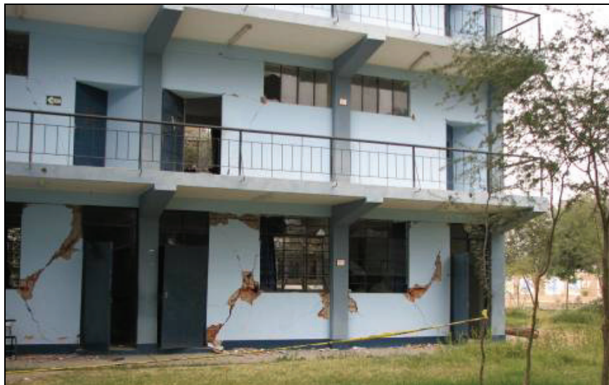
Figure 6.33 Damaged infill walls of a building at the National University of Ica
