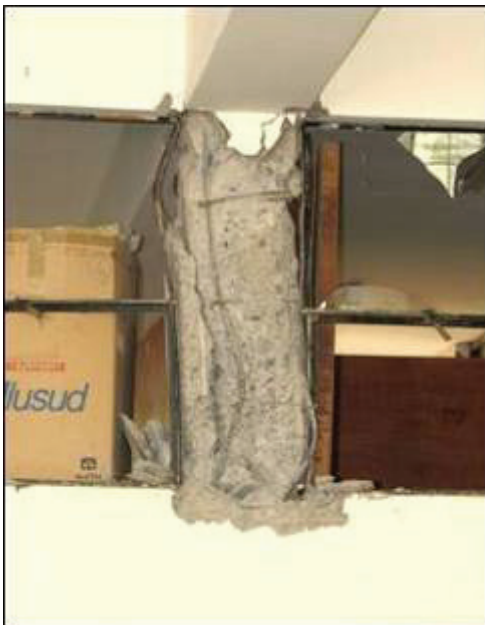
(e) Shear failure, CW11
