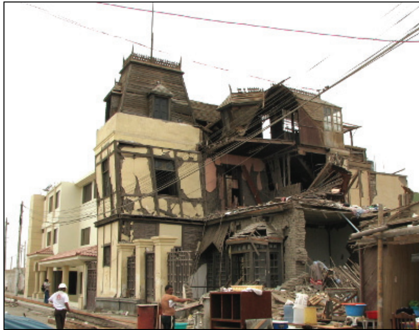
Figure 6.3 Residential building made of reinforced adobe-1
