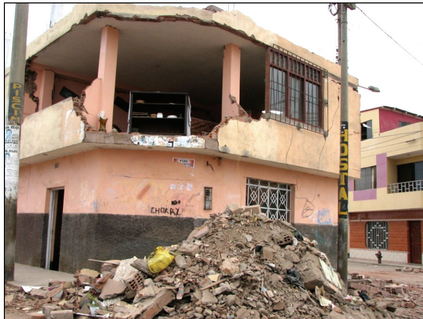
Figure 6.55 Out-of-plane failure of infill walls in Ica
