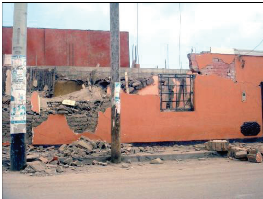
Figure 6.10 Collapsed masonry structure-4
