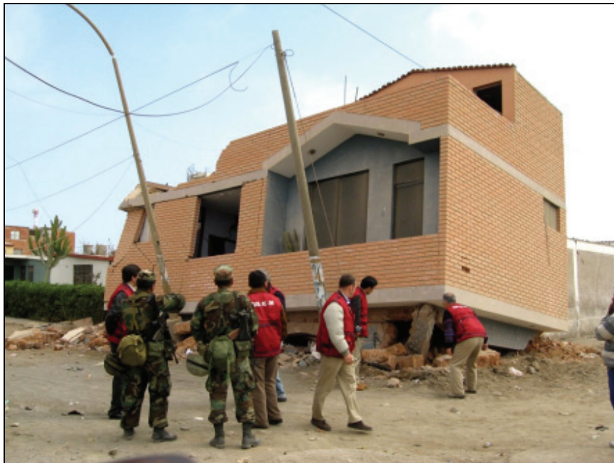
Figure 6.12 Collapsed masonry structure with RC columns-6
