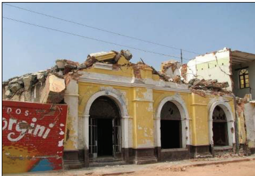
Figure 6.8 Collapsed masonry structure-2
