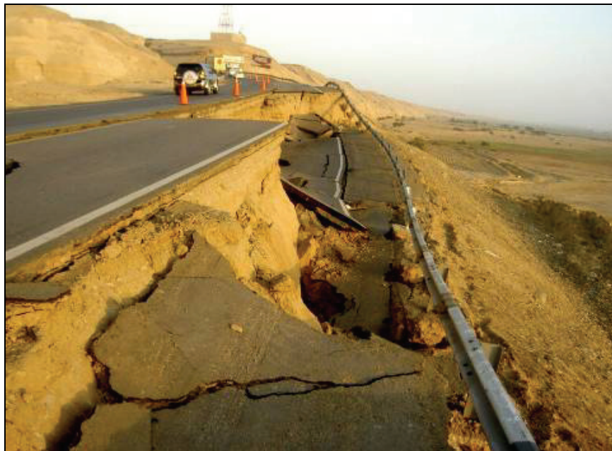
Figure 6.46 Road failure from slope failure
