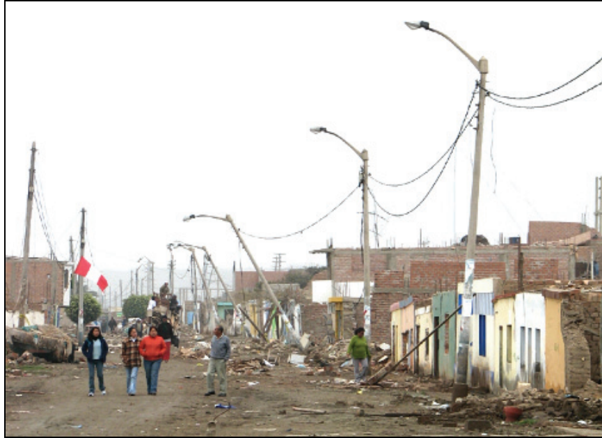
Figure 6.28 An area where most buildings were damaged due to liquefaction
