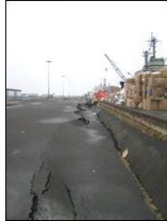
b) Vertical displacement of 80 cm
