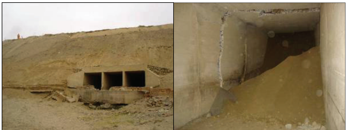
a) View of a concrete sewer under the embankment
