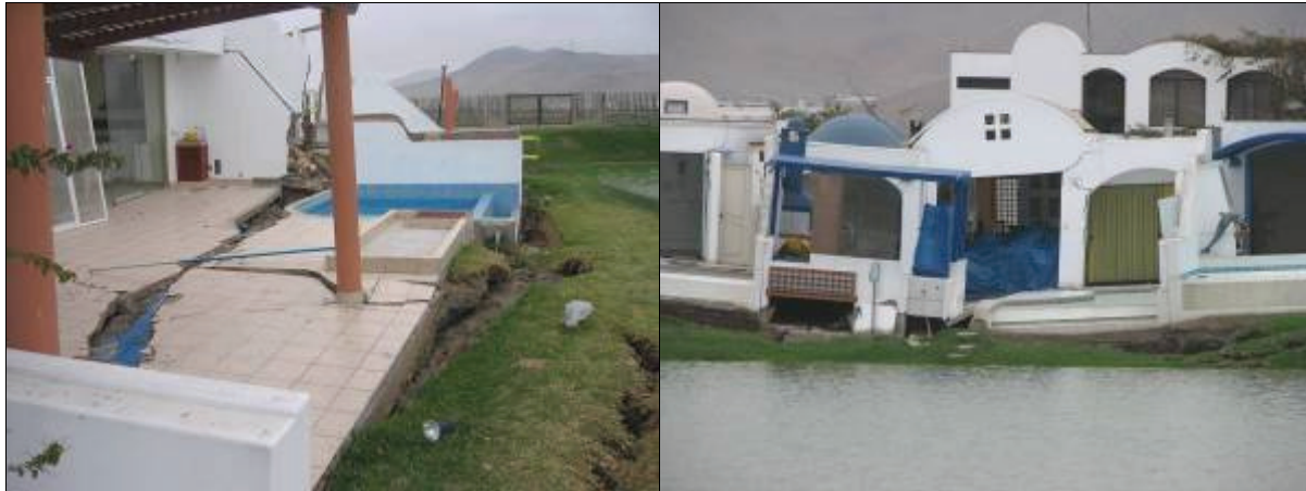
a) Settlement of houses next to the lakeshore b) Cracks in houses due to soil displacement Figure 5.7 Damage in Las Lagunas at 70.5 km along the Pan-American South highway
