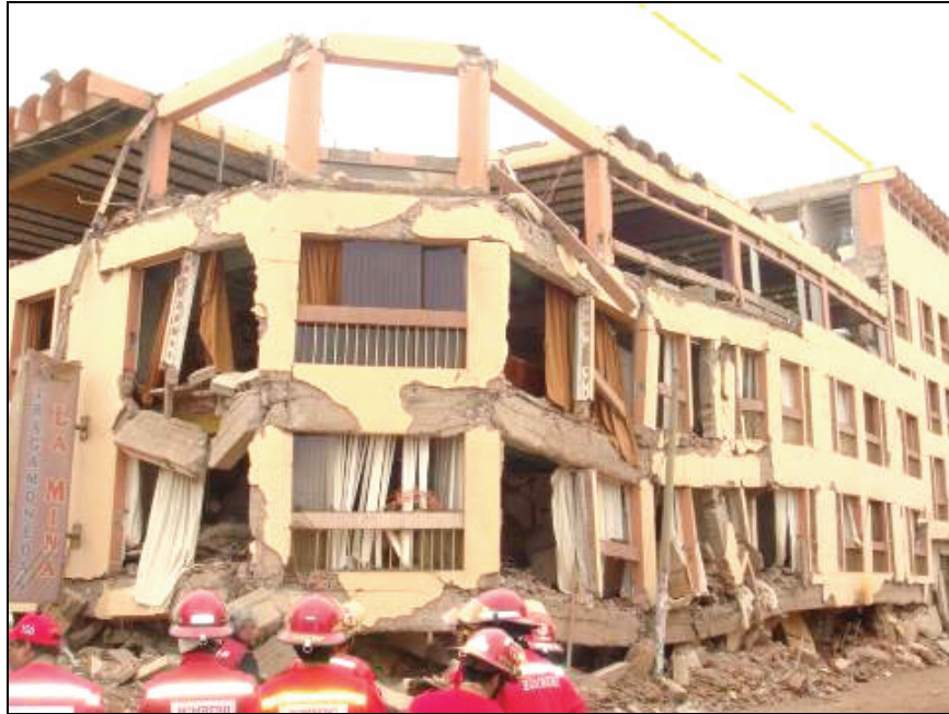
Figure 6.15 Soft story collapse of RC structure-3
