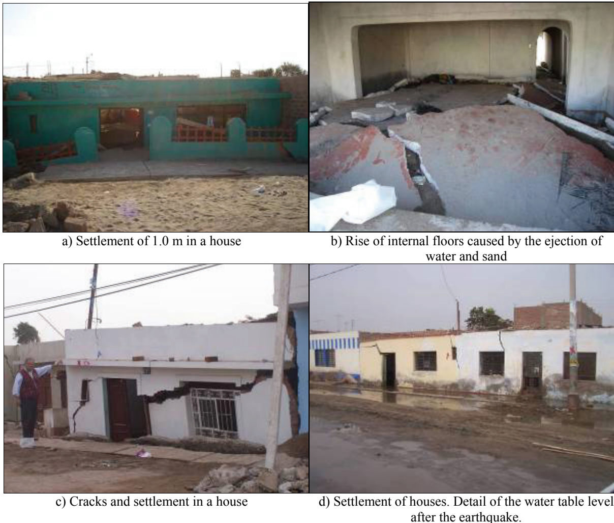
Figure 5.3 House damage caused by the settlement of foundations. Alfonso Ugarte Street in Tambo de Mora District
