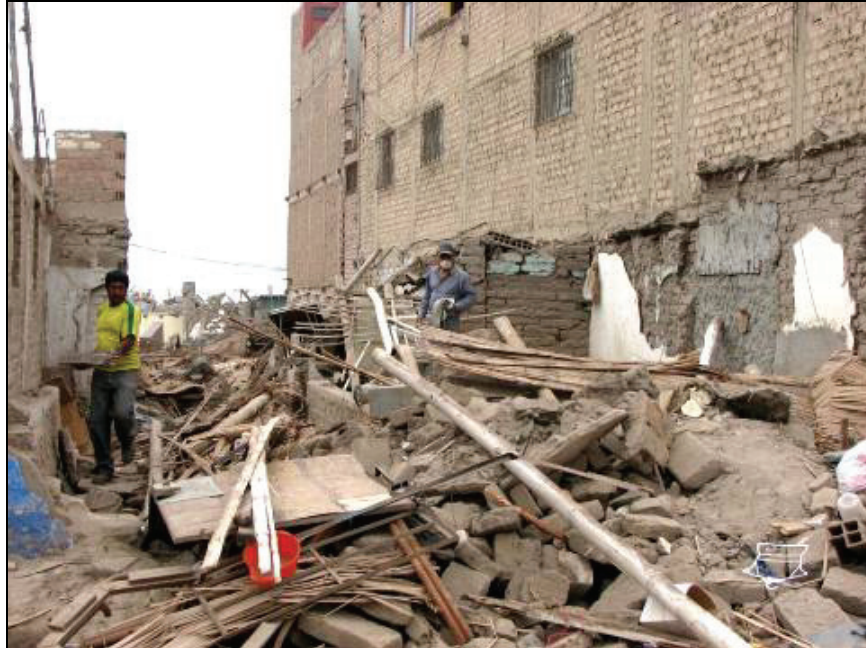
Figure 6.9 Collapsed masonry structure-3
