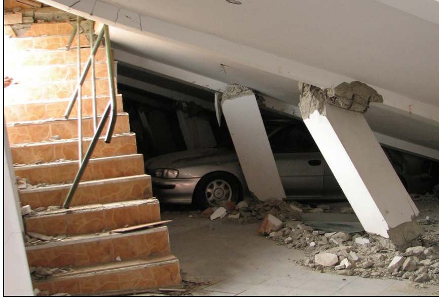
Figure 6.54 View of inner columns of collapsed building at Pisco Playa
