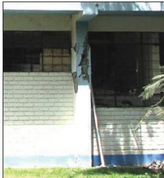
(b) Shear failure, CW18
