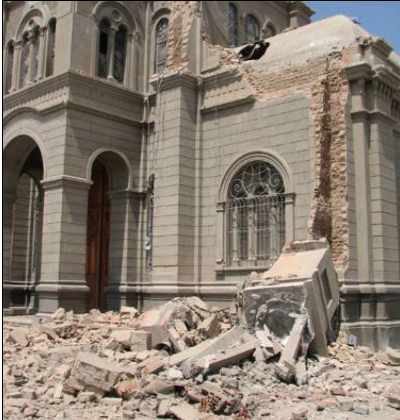
Figure 6.36 Collapse of massive masonry church building
