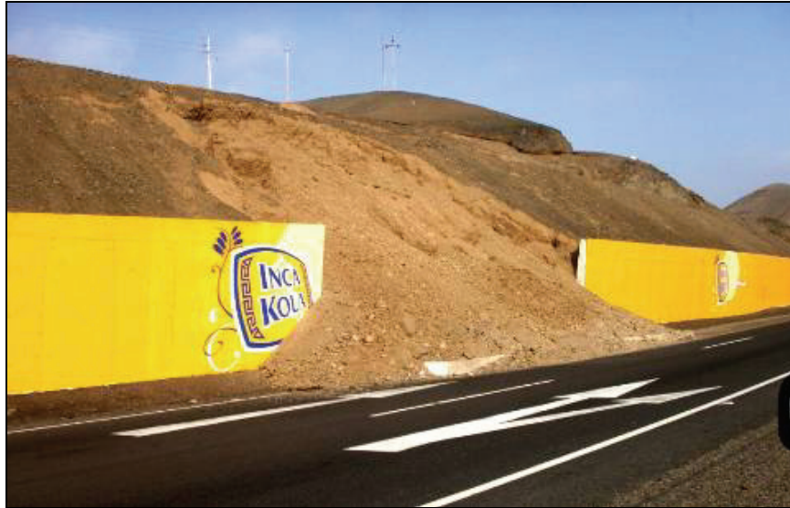
Figure 6.43 Slope failure and damage to highway
