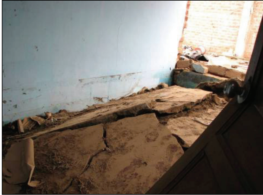
Figure 6.30 Upheaval of floor slabs
