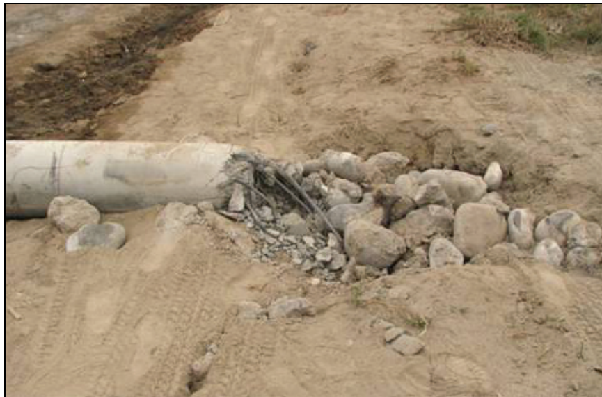
Figure 6.38 Collapse of power transmission structure - structural failure
