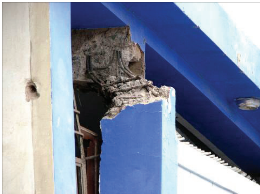
Figure 6.18 Shear failure of beam-column connection close-up
