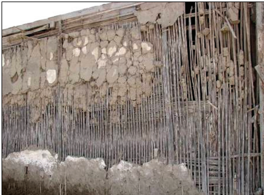
Figure 6.6 Typical layout of reinforcement and adobe of residential building
