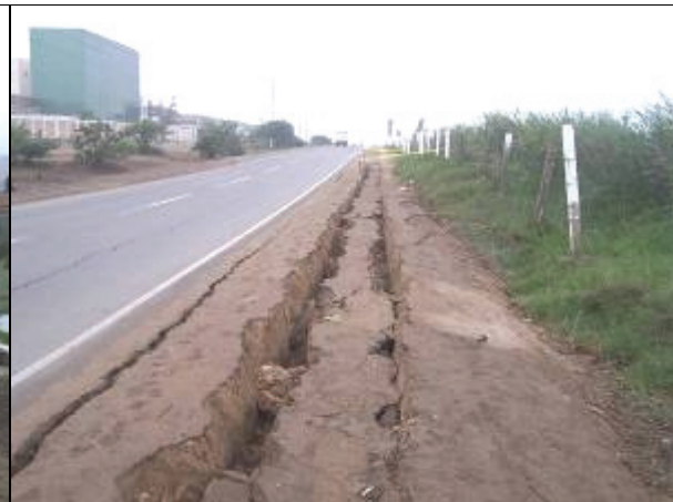
b) Cracks in the pavement and berm of the highway
