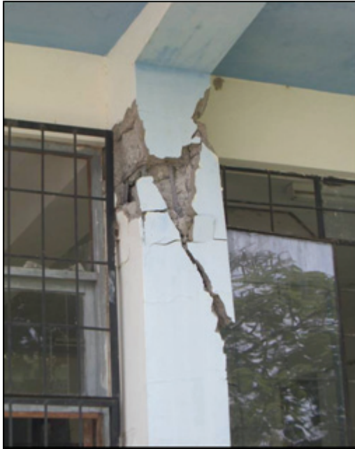
(c) Shear failure, CW03
