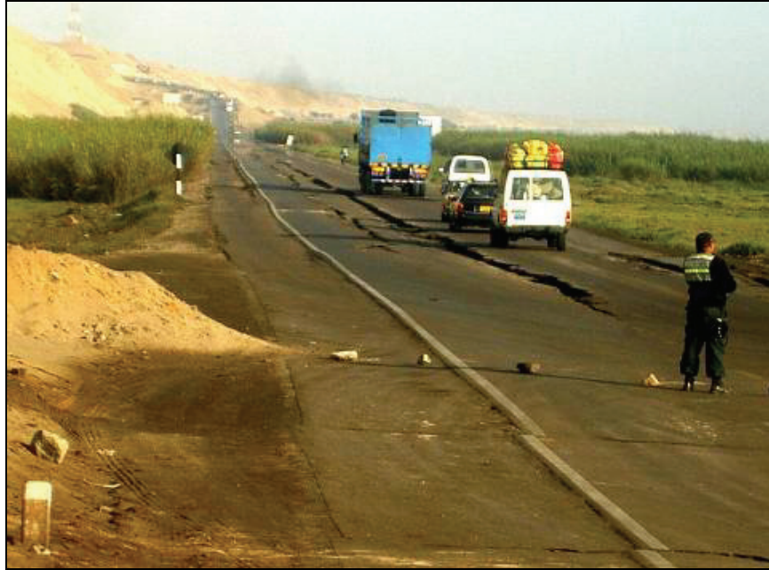
Figure 6.45 Road failure from lateral spreading parallel to the road
