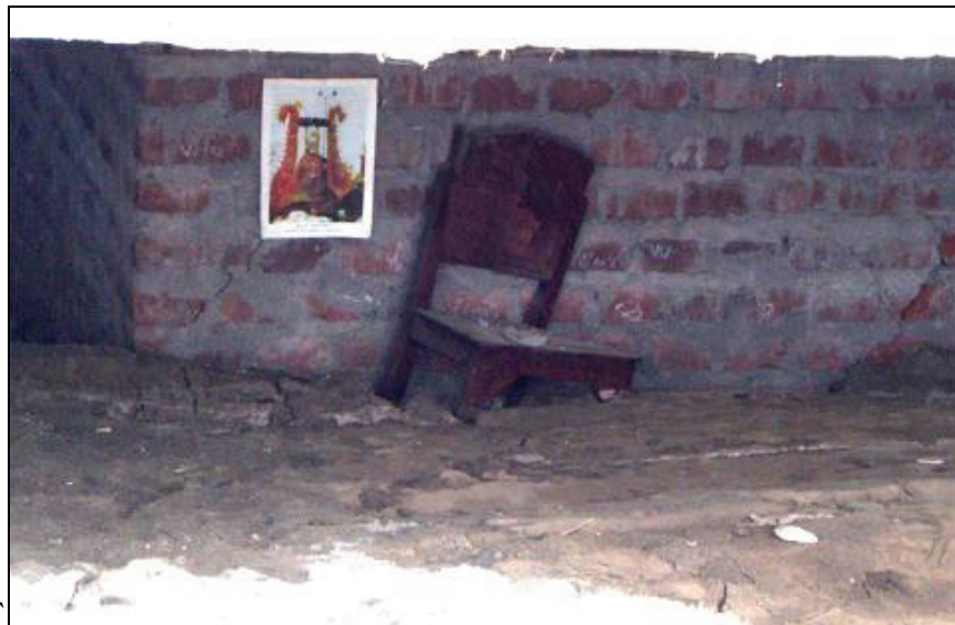
Figure 6.31 A chair partially buried in liquefied soil
