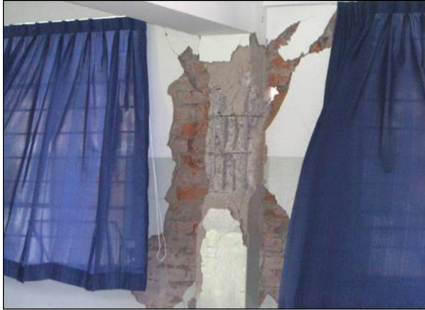
Figure 6.34 Shear failure of a column at the National University of Ica
