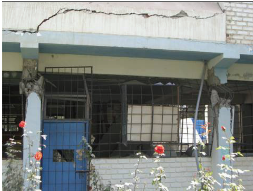
Figure 6.35 Failure of columns of a building at the National University of Ica
