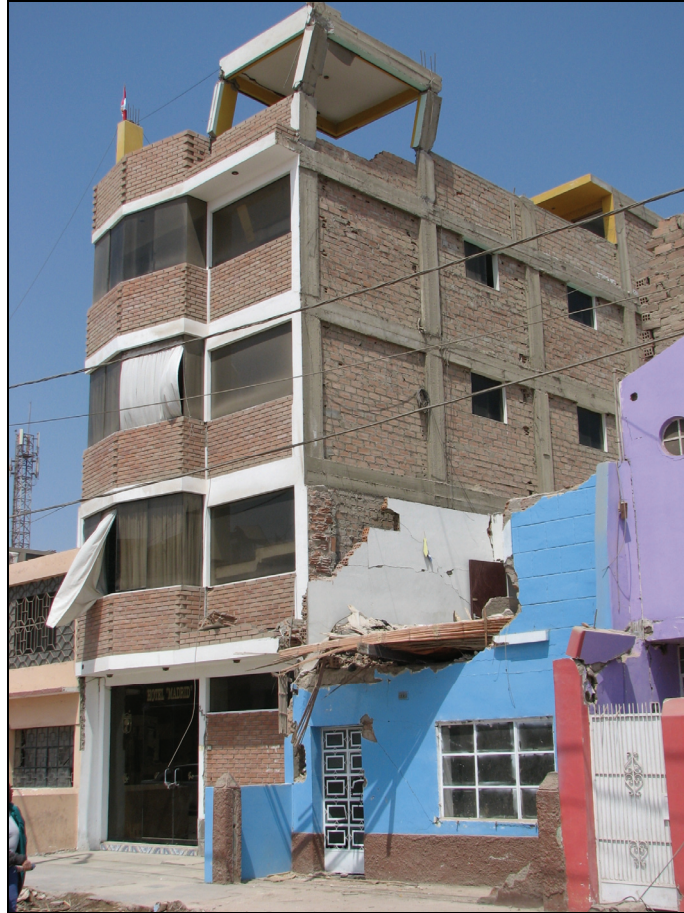
Figure 6.59 Added element about to fall down from the top floor of a building in Pisco.
