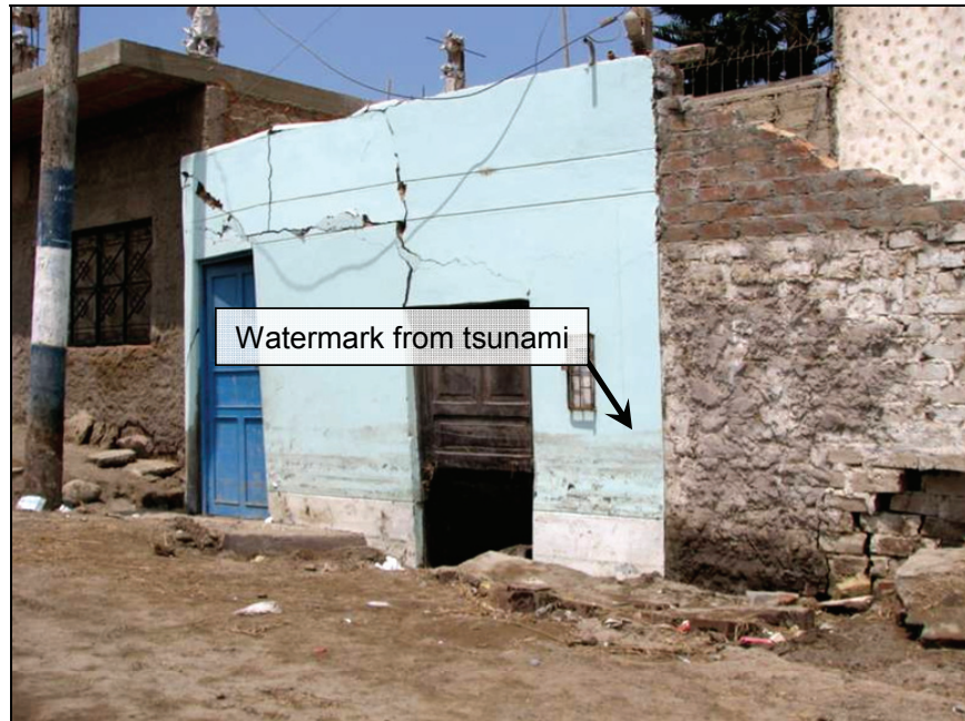
Figure 6.25 Buildings with watermarks from tsunami-1
