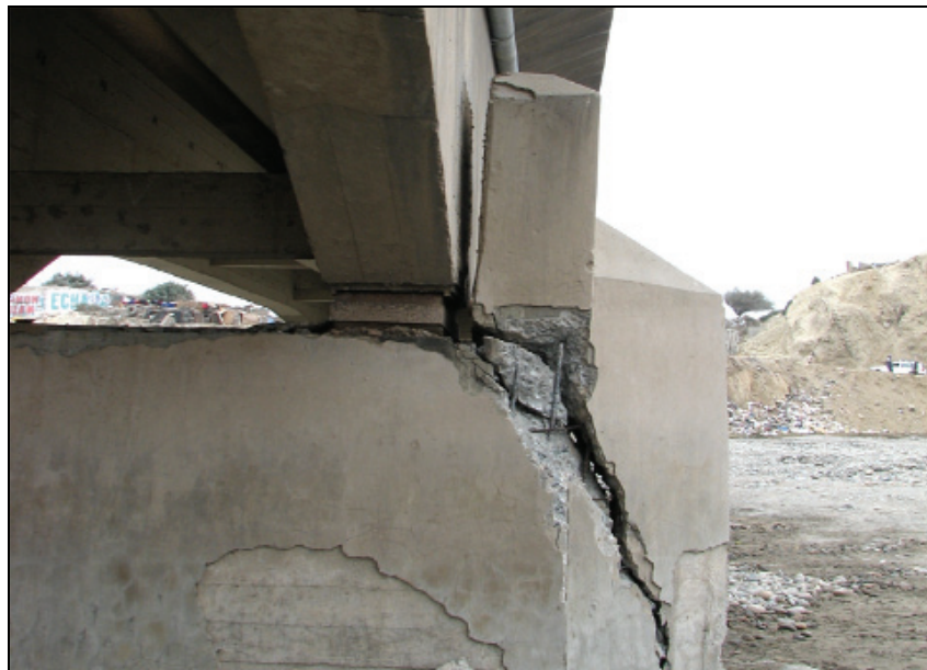
Figure 6.48 Damage to shear key of a bridge
