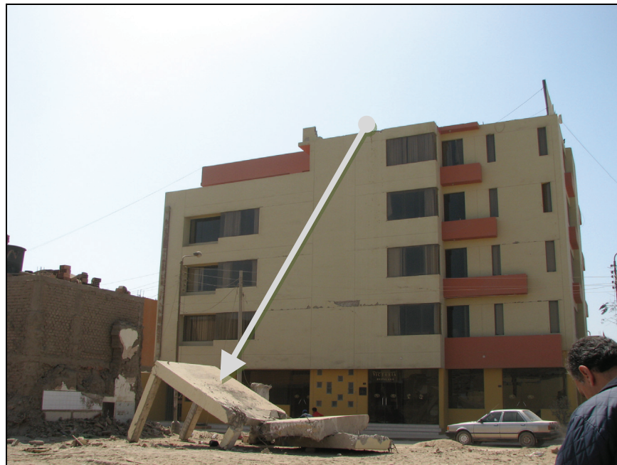
Figure 6.58 Collapse of an extension from the top floor of a building in Pisco
