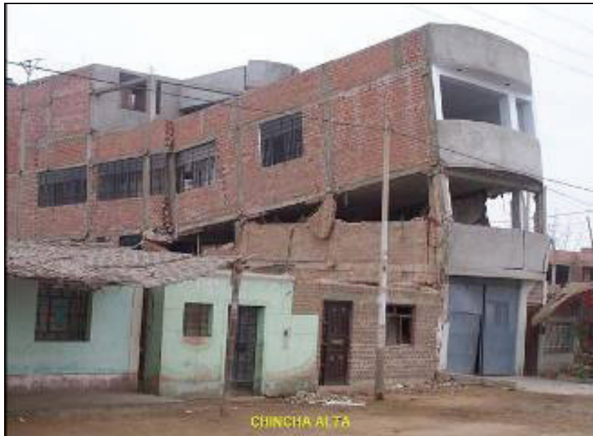
Figure 6.52 Failure of a three-floor building in Chincha Alta due to intermediate soft story
