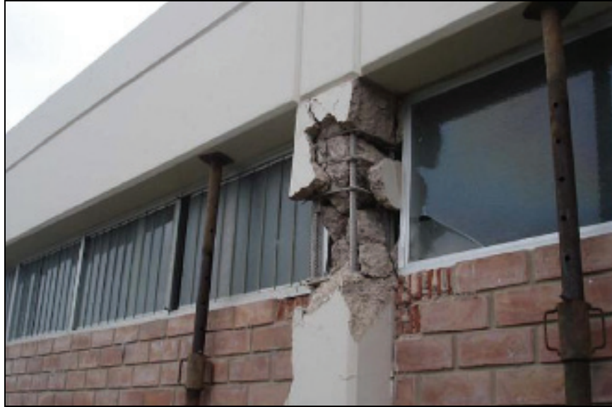
Figure 6.49 Short column failure at office building in Pisco
