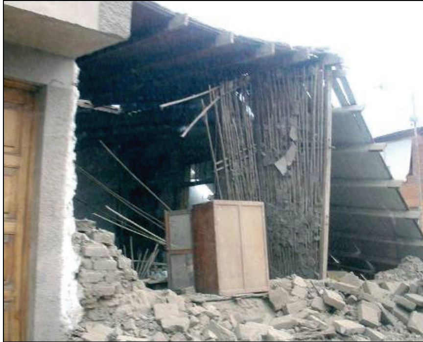
Figure 6.5 Adobe wall supporting roof
