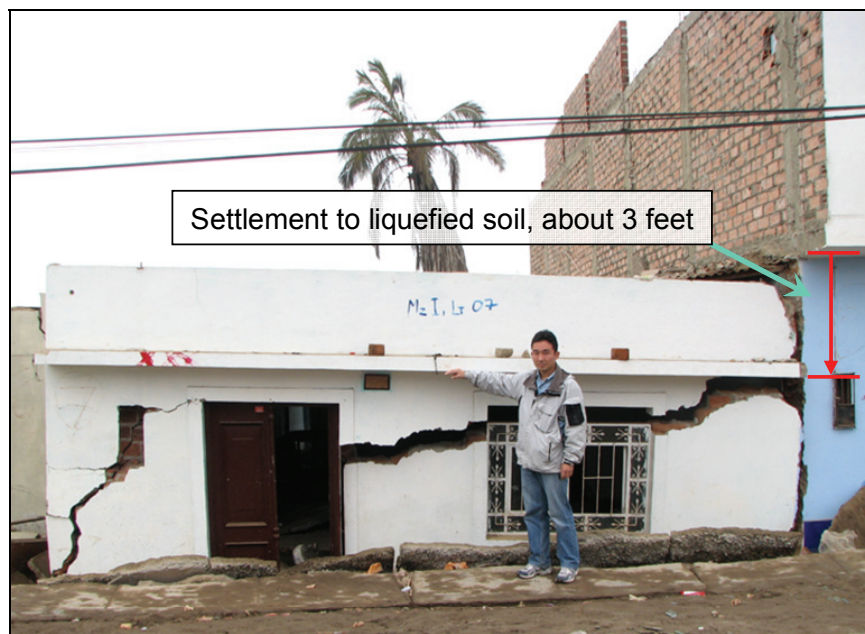
Figure 6.29 Masonry building that sunk 3 feet due to liquefaction
