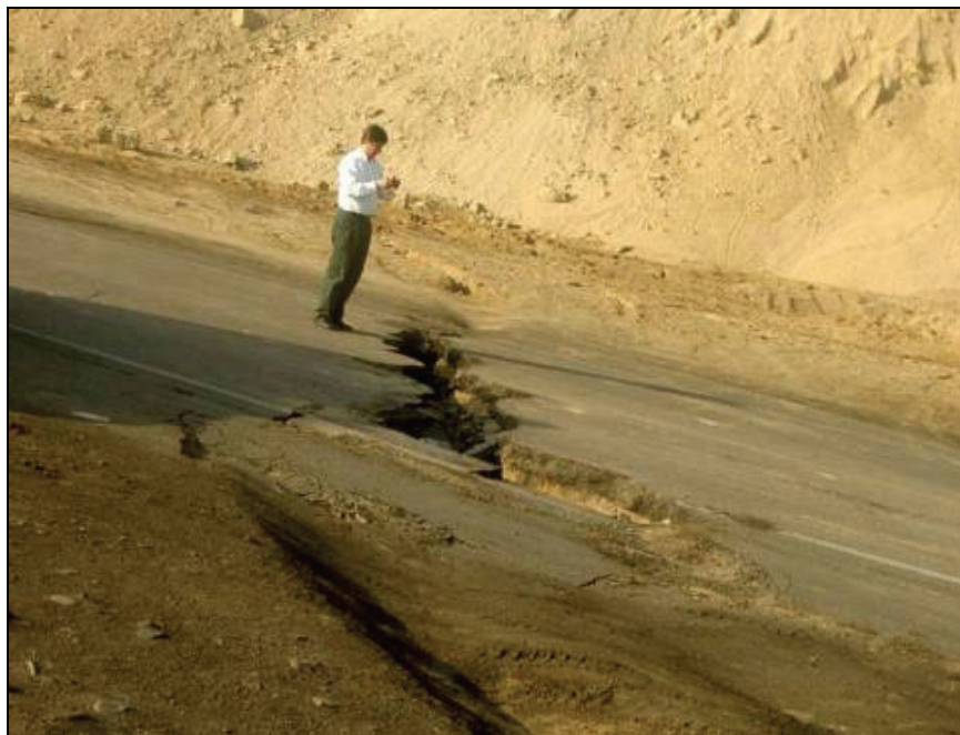
Figure 6.44 Road failure from lateral spreading perpendicular to the road
