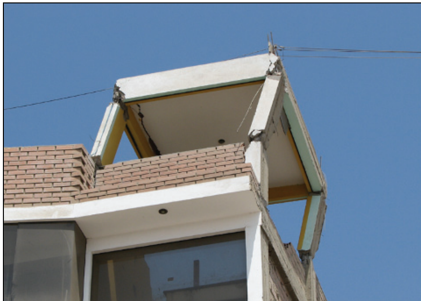
Figure 6.20 Failure due to short column effect from masonry infill wall
