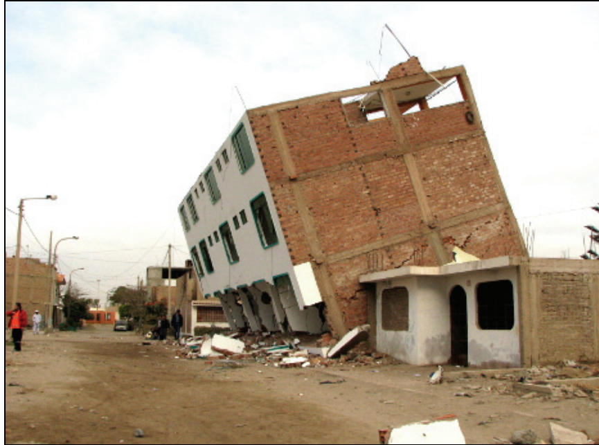
Figure 6.13 Soft story collapse of RC structure-1
