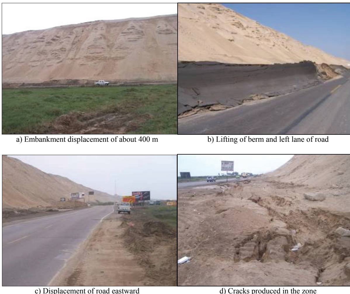
Figure 5.8 Soil displacement in the Jahuay in the 188 km of the SPA Highway caused by liquefaction in the slope foot
