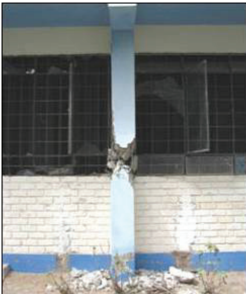
(a) Moment-axial interaction failure, CW16
