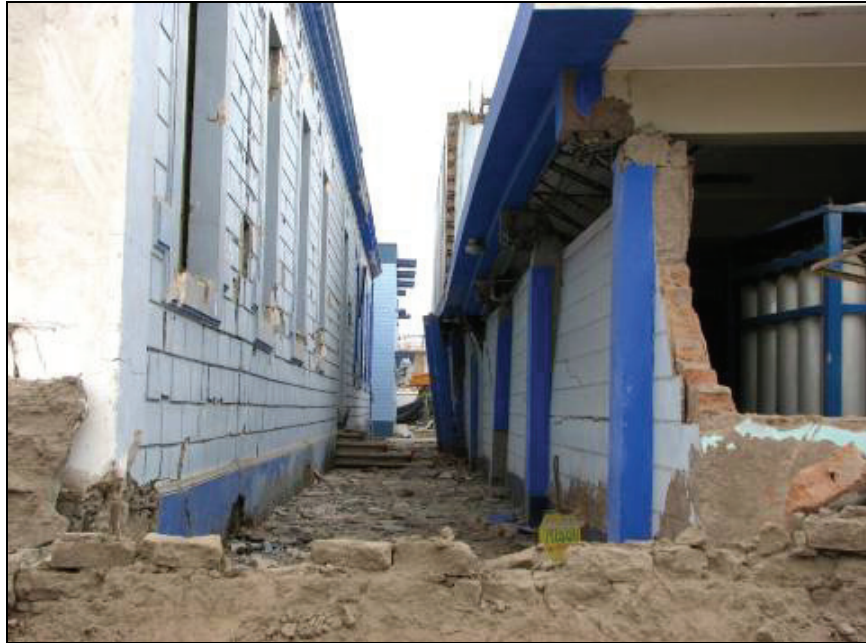
Figure 6.17 Shear failure of beam-column connection
