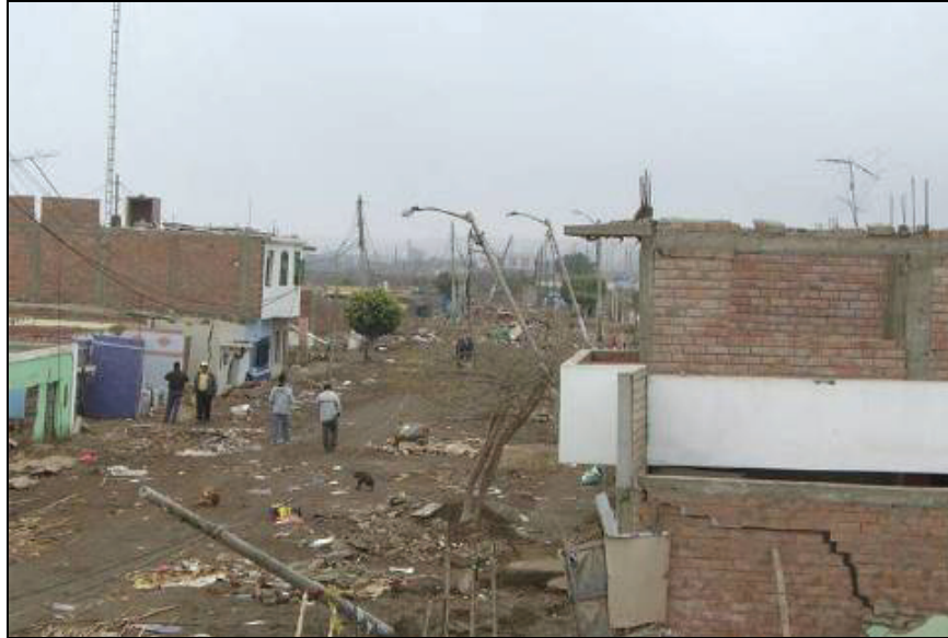
Figure 6.41 Collapse of power transmission lines
