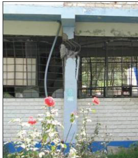
(f) Shear failure, CW06
