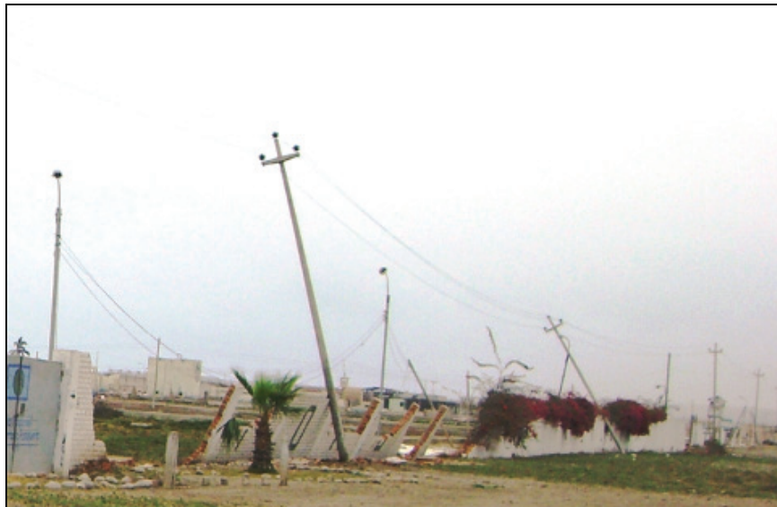
Figure 6.40 Tilting power transmission lines - foundation failure
