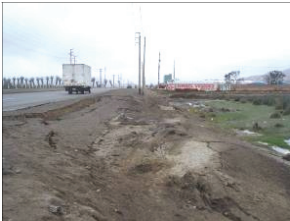
a) Ground displacement due to soil liquefaction
