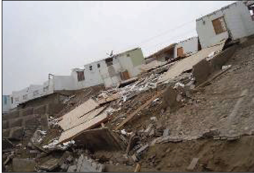
Figure 6.60 Collapsed buildings due to slope instability
