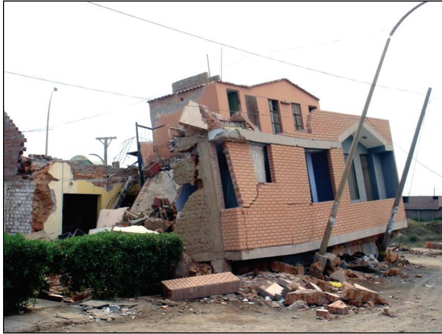
Figure 6.51 Collapse of housing unit in Pisco due to soft story problems
