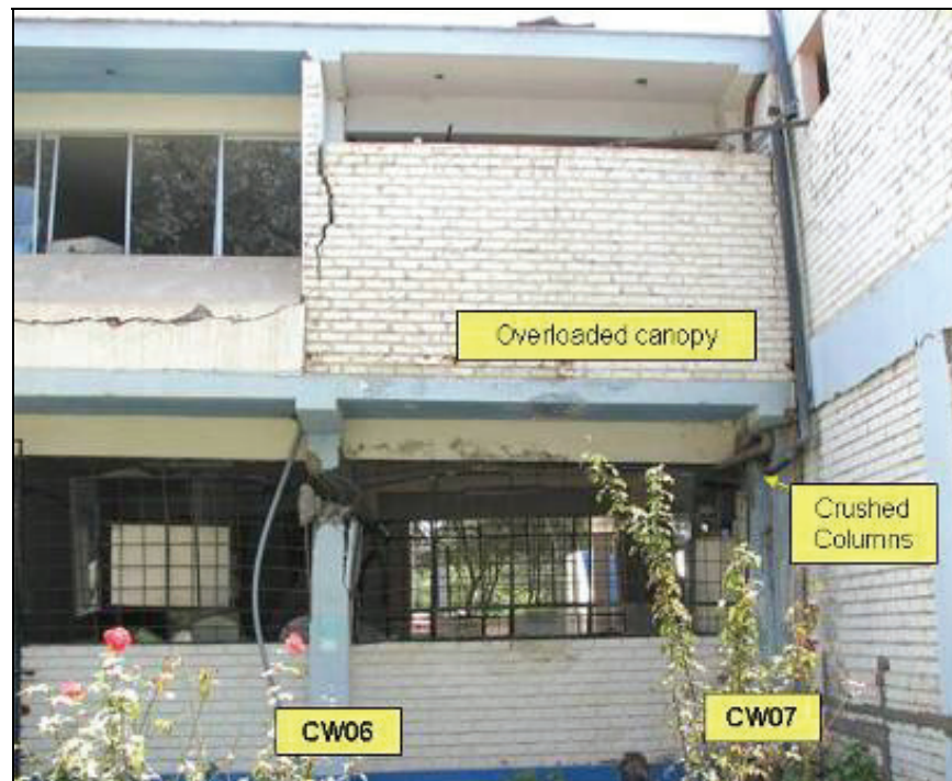
Figure 7.8 Overloaded span of the building
