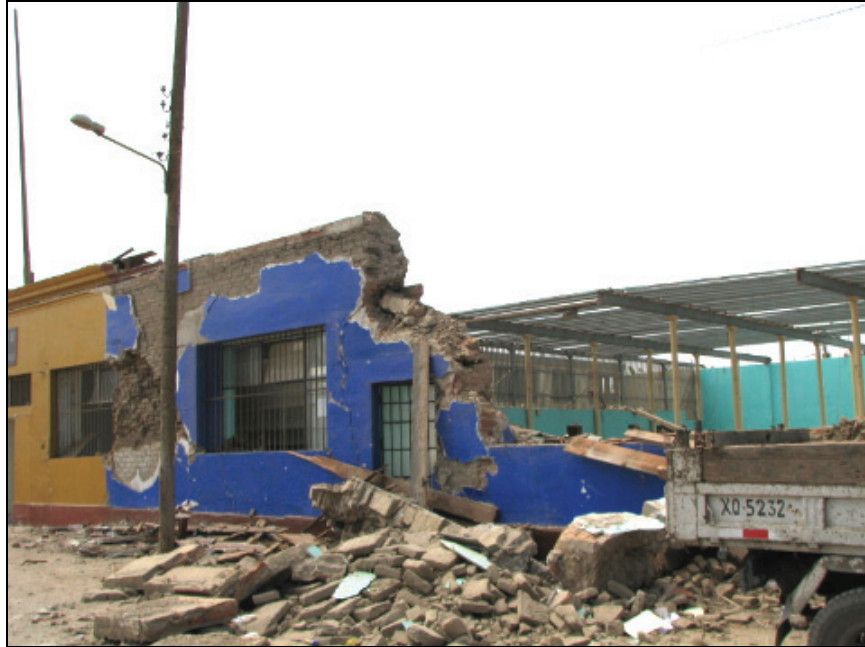
Figure 6.7 Collapsed masonry structure-1
