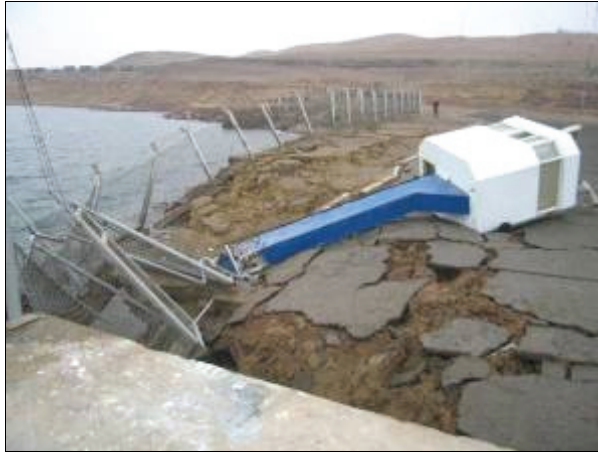
a) Structural collapse due to ground cracks in areas gained to the sea
