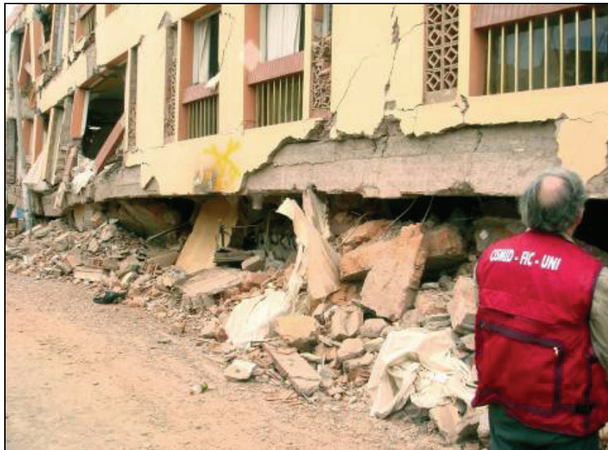
Figure 6.16 Soft story collapse of RC structure-3
