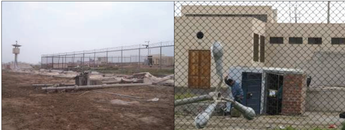
a) Collapse of walls and high-voltage poles
