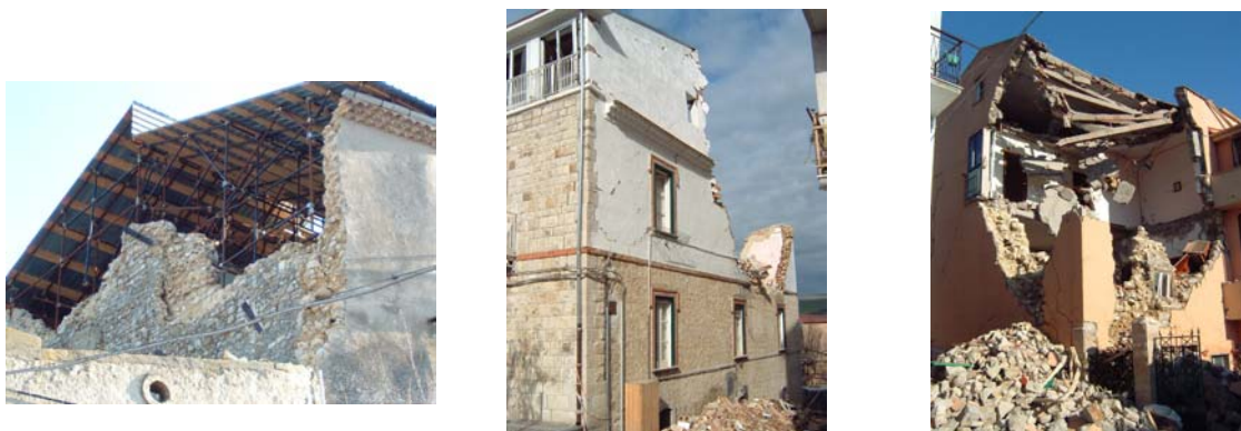
Figure 7.10. Out-of-plane damage patterns
