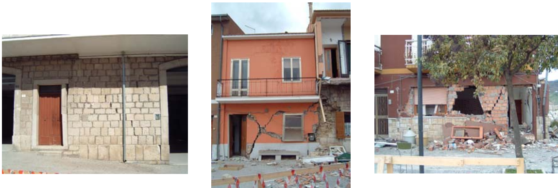
Figure 7.9. In-plane damage patterns, bed-joint-sliding and diagonal cracking
