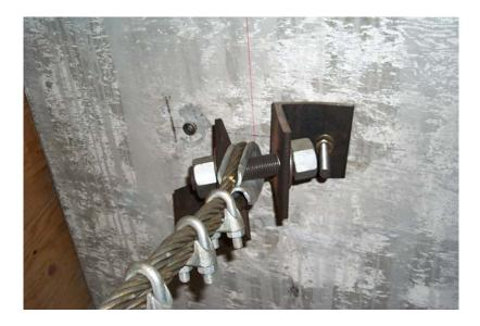
Figure 7.56 Failure of undercut anchor at pier connection in retrofit modification 4.
