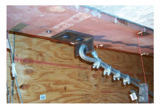
Figure 7.37 L8x4x1/2" steel angle used at the girder connection as part of retrofit modification 1.
