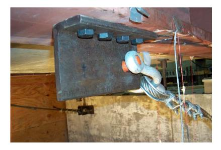
Figure 7.63 View of girder connection showing bolts and shackle.
