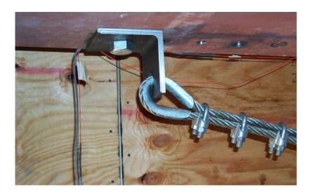
Figure 7.43 L6x6x1/2" steel angle used at girder connection in retrofit modification 2.
