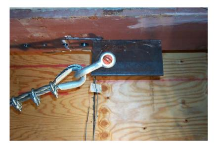
Figure 7.62 Side view of girder connection used in retrofit modification 6.
