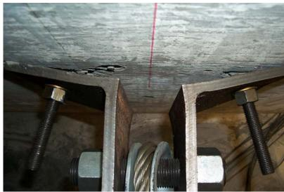
Figure 7.55 Damage due to prying action of pier connection.
