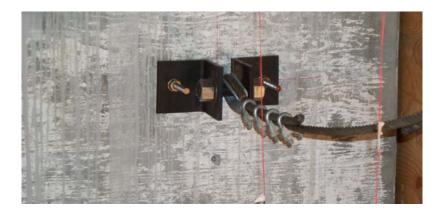
Figure 7.42 Two L6x6x1/2" steel angles back-to-back used in retrofit modification 2.
