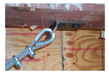
Figure 7.40 Angle girder connection used in retrofit modification 1 with ductile deformation.
