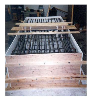
Figure 7.3 Reinforcement cage and form for the construction of the piers.
