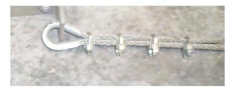
Figure 7.13 Wire rope end termination used a thimble and 4 wire rope clips.
