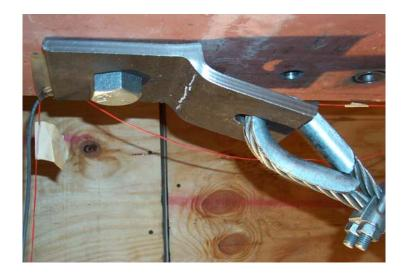
Figure 7.45 Angle connection at girder used in retrofit modification 2.
