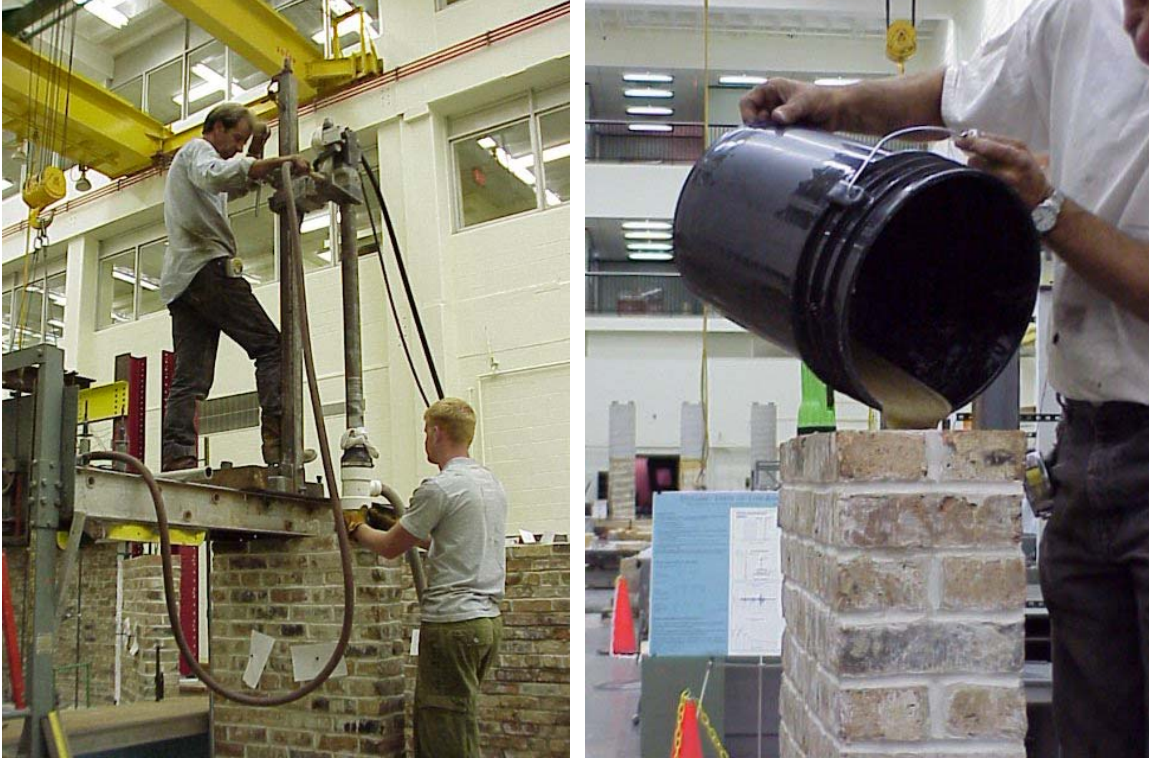
Figure 2-11 Drilling of Cores and Placement of Epoxy-Grout
