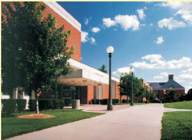
Newmark Civil Engineering Laboratory
